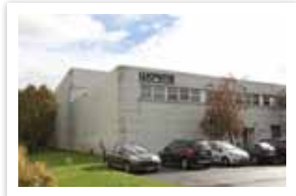
IMER France - WORMS Entreprises (Power Generators) Paris, France
